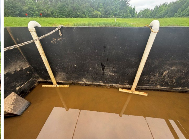
(b) water delivery system
