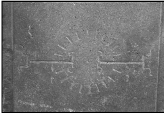
Figure 18 Encircled Hooked Bars.
