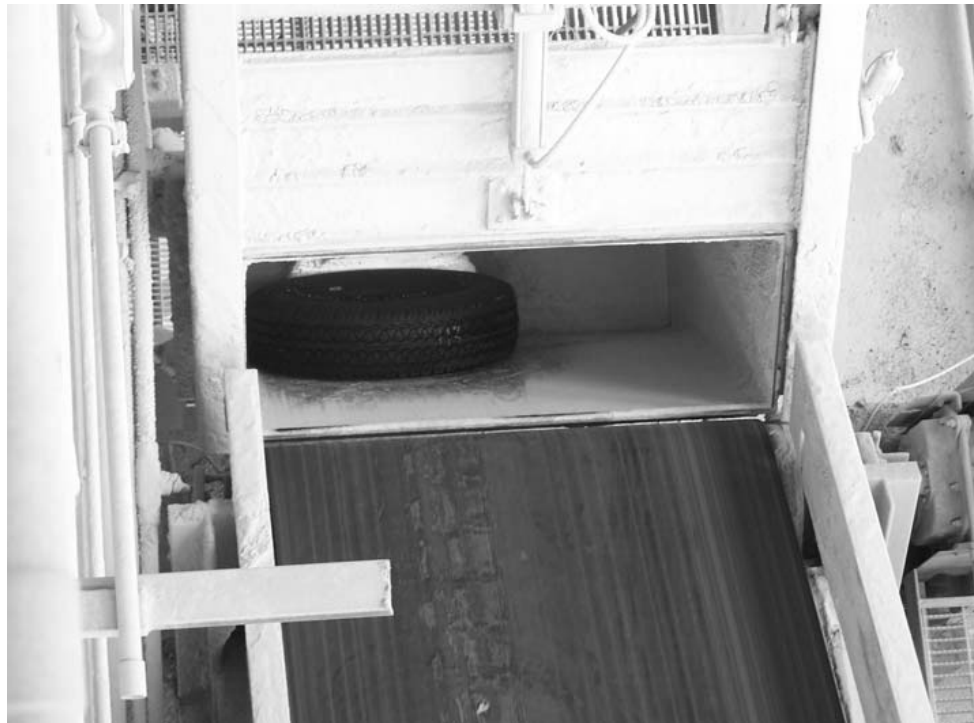
Figure 3.8: Tires entering kiln through drop chamber
