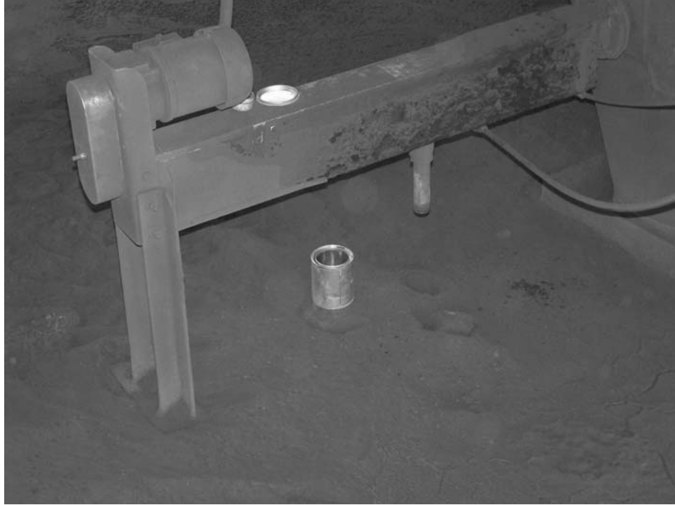
Figure 3.6: Automated plunger system collecting coal/coke samples
