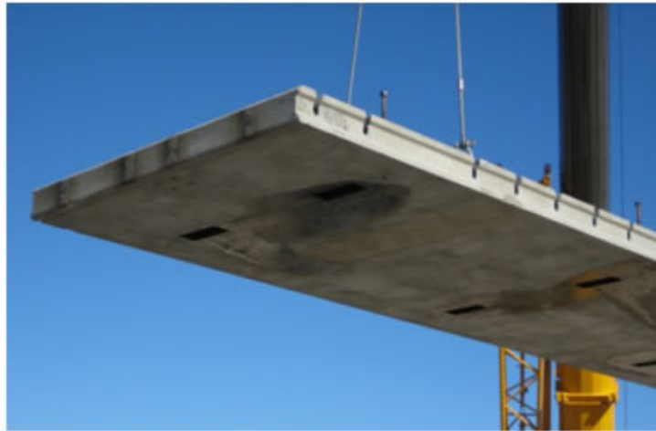
Figure 1.3: Typical Full-Depth Precast Panel (Culmo 2000)
