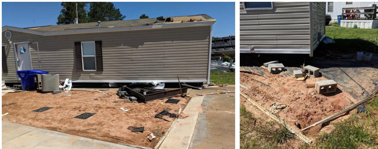
Figure 4-21. MMH lifted and rotated off of foundations
