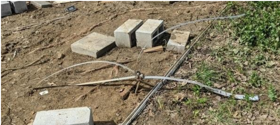
Figure 4-23. Failed strap system with multiple apparent connections
