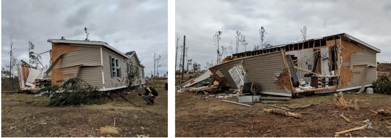
Figure 4-2. Failure at the marriage line
