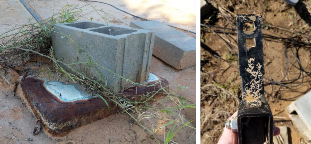
Figure 4-15. Failure mechanisms of a Xi2 pan system
