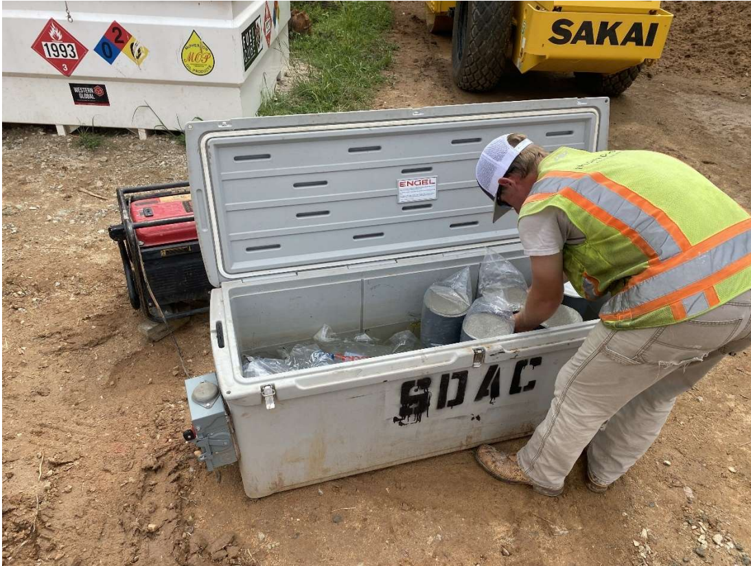
Figure 4-27: Jobsite 4 Contractor Curing Box
