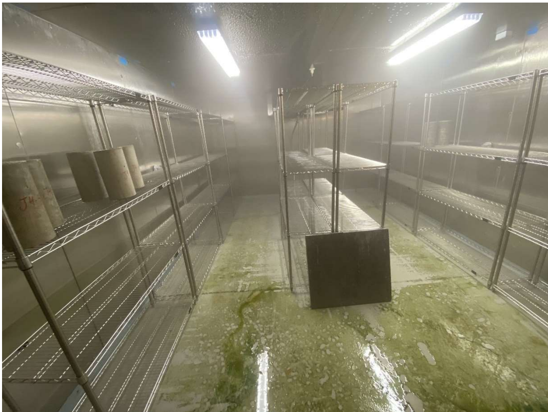
Figure 3-5: Final Curing Room
