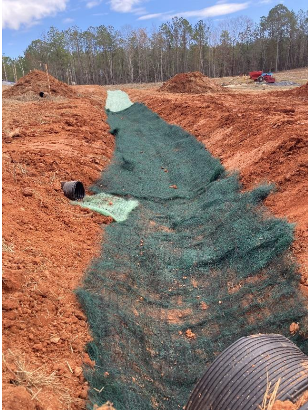
(a) TRM installation
