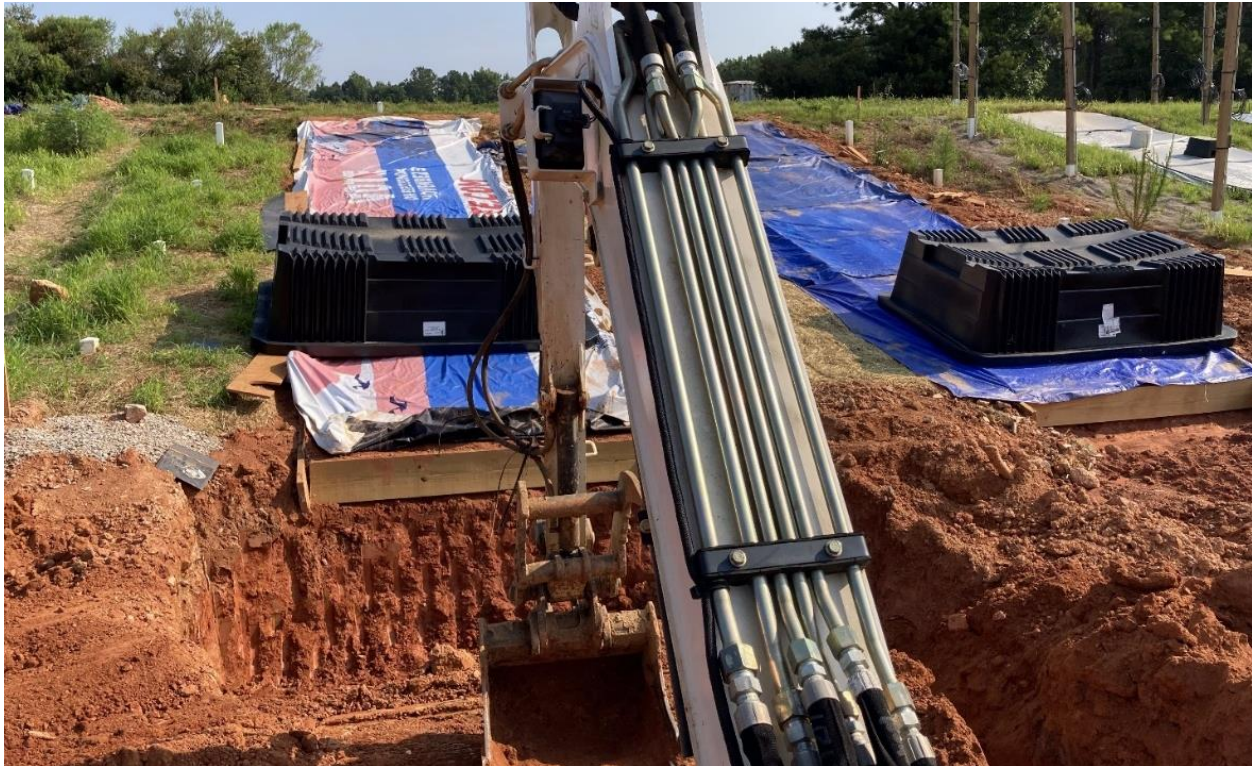
FIGURE 3.9: Excavation for Catchment Basin and Anchoring.
