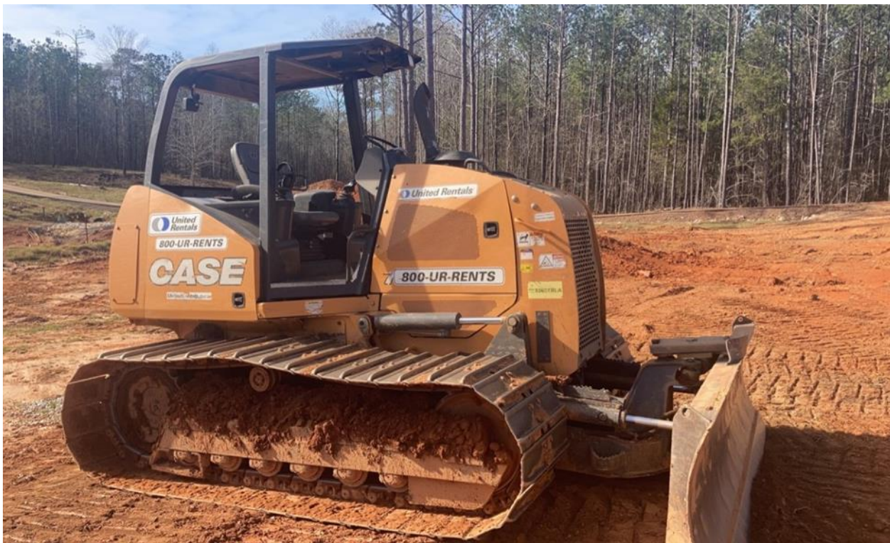
FIGURE 3.5: Bulldozer for Regrading.
