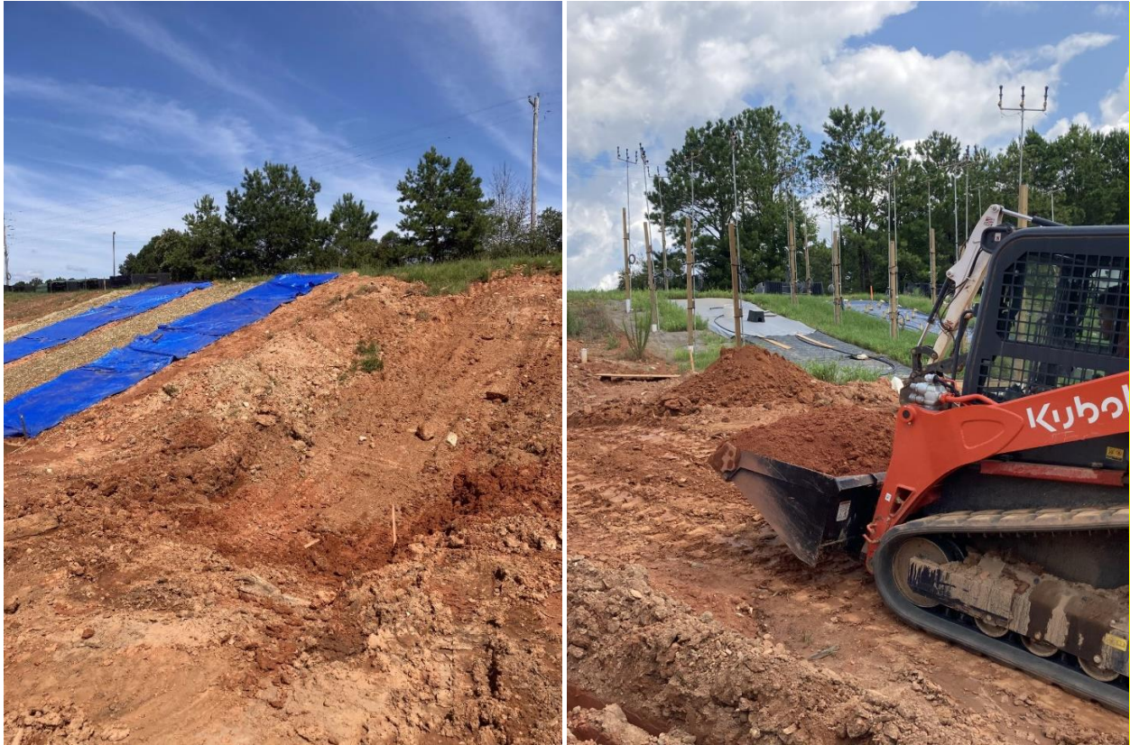
(a) Plot 8 excavation
