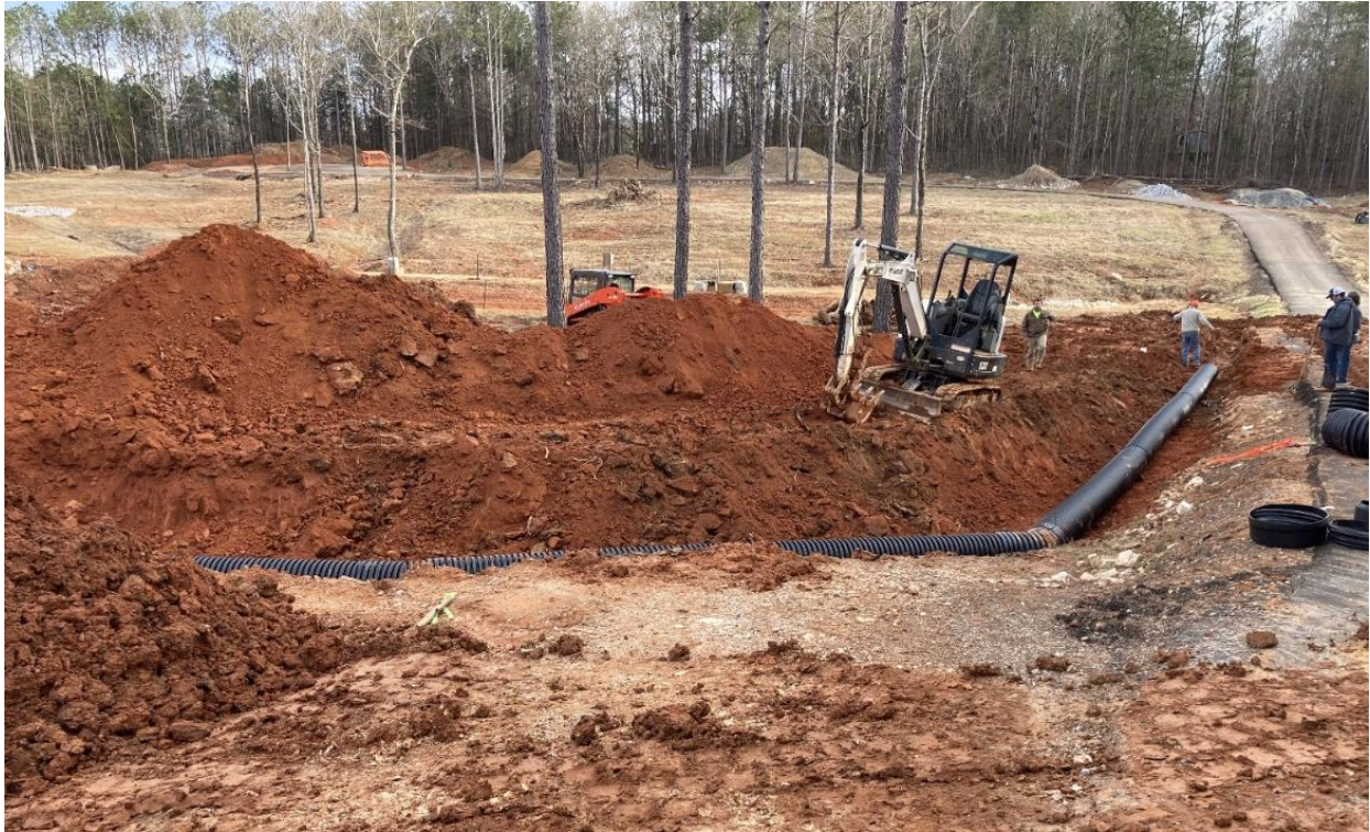
FIGURE 3.11: Drainage Pipe Installation.
