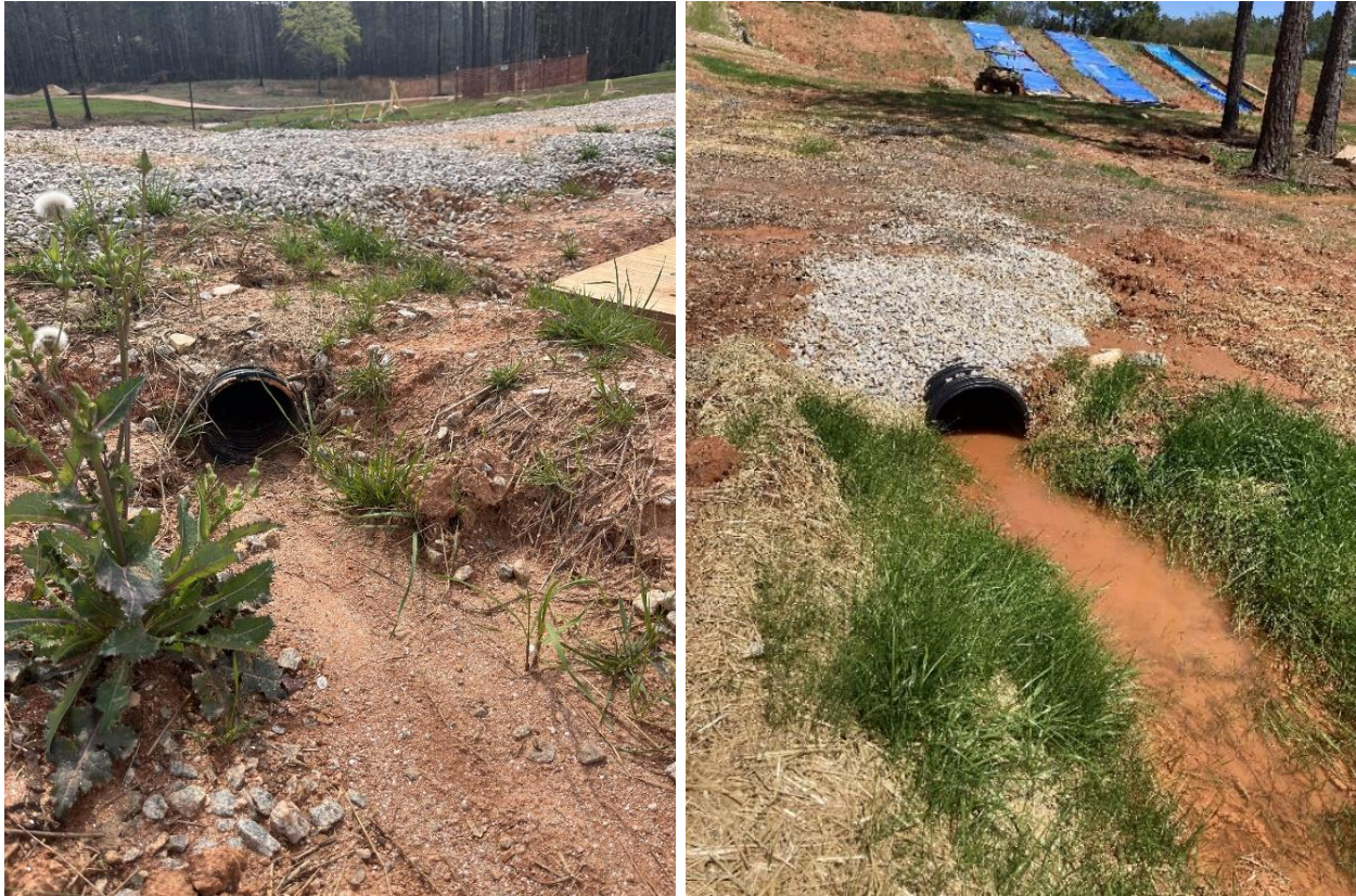
(a) Plot 7 culvert
