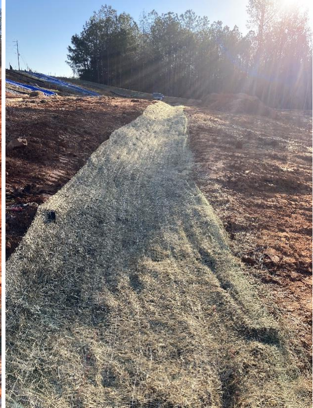
(b) ECB installation
