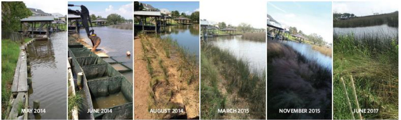
Figure 2.6 Project locations (Top) and progression photos of a living shoreline at location C in Mobile Bay (Bottom) (TNC, 2023)
