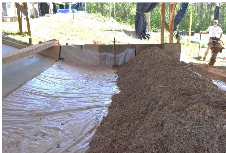
Figure 3: Updated Slash Mulch Berm Installation, Offset from Toe of Slope
