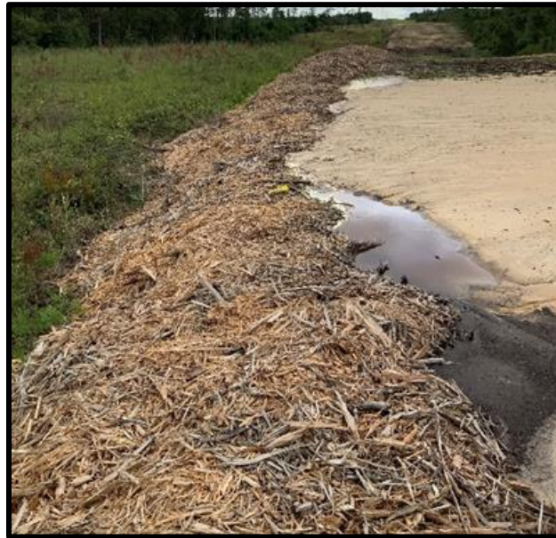
Figure 3.5 Slash Mulch Berm Installation (photo courtesy of Cliff Young 2021)
