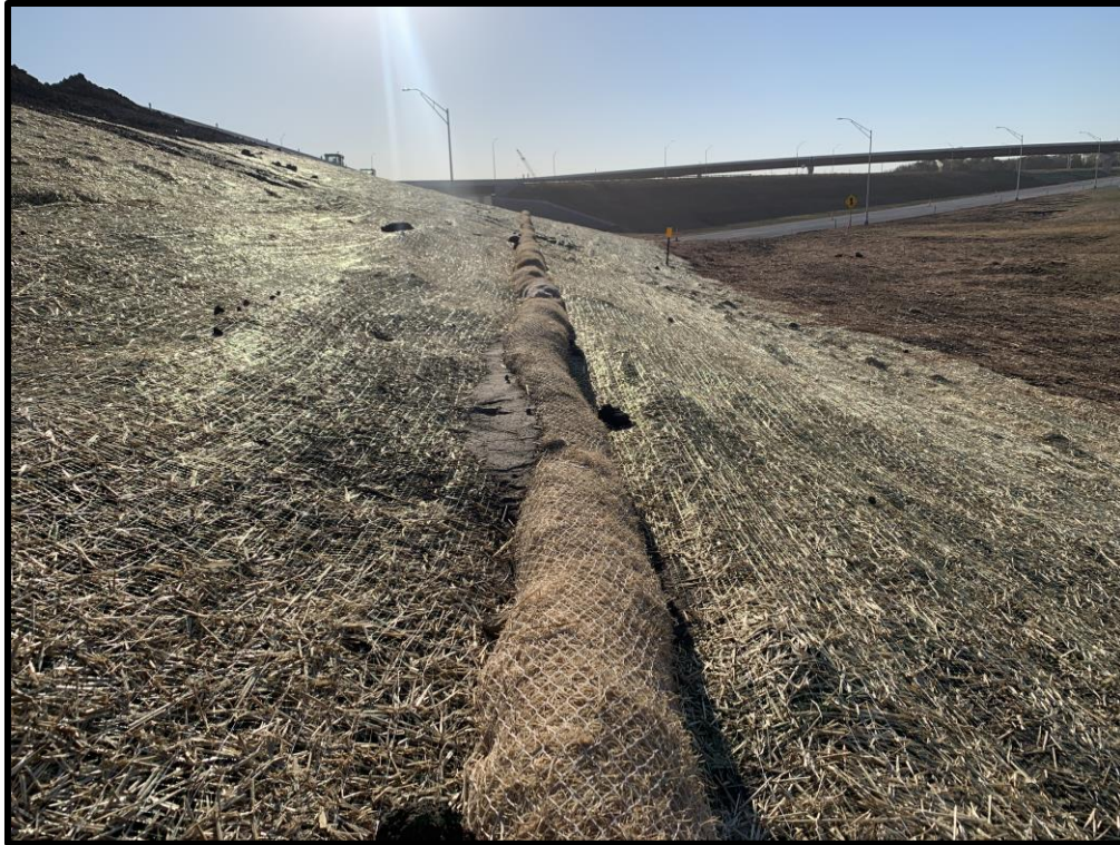
(a) wattle as slope protection
