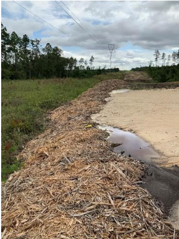
(a) installed slash mulch berm
