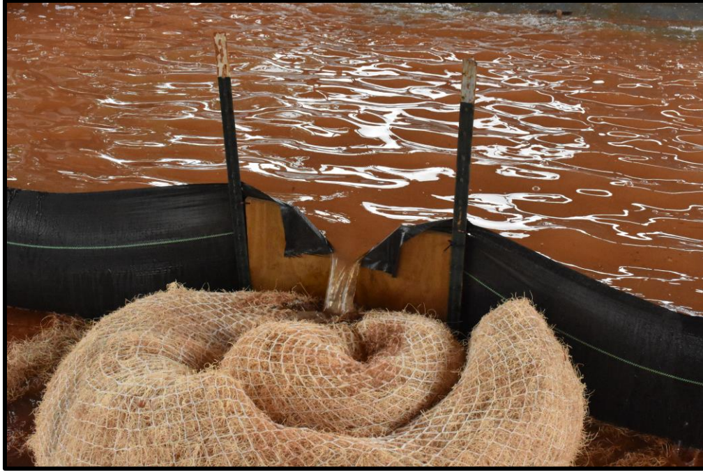
Figure 3.16 Overflow Weir Dewatering
