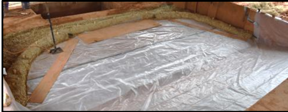
(a) straw wattle standard installation
