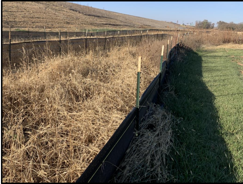
Figure 3.1 Nebraska DOT Silt Fence Installation
