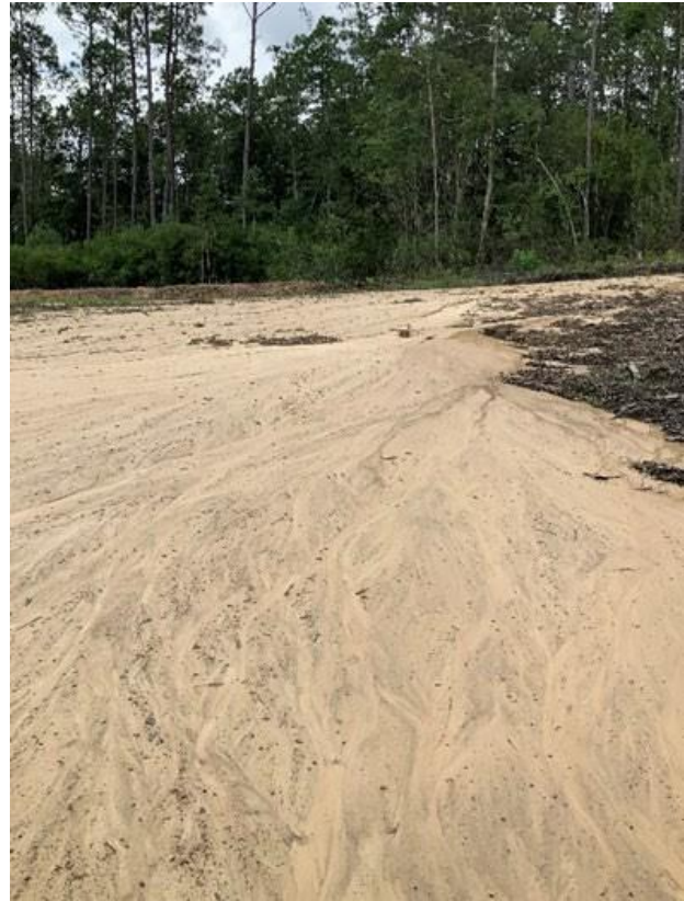
(b) sedimentation upstream of berm
