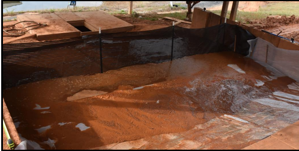
Figure 3.18 Performance of High Porosity Silt Fence Installation
