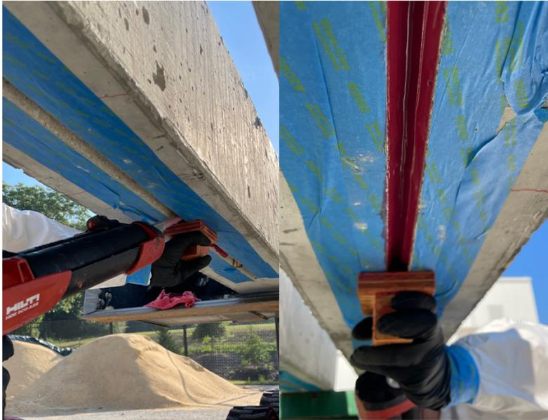
**Figure 7.12— First Lift of Epoxy application**
