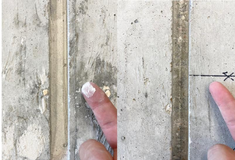
**Figure 7.11— Before (Left) and After (Right) Water Blasting with Abrasives**
