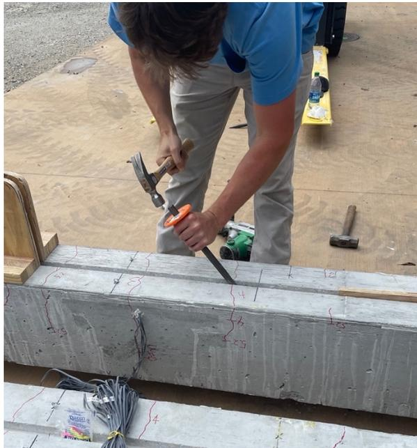
**Figure 7.9— Chiseling to Refine Bevel**
