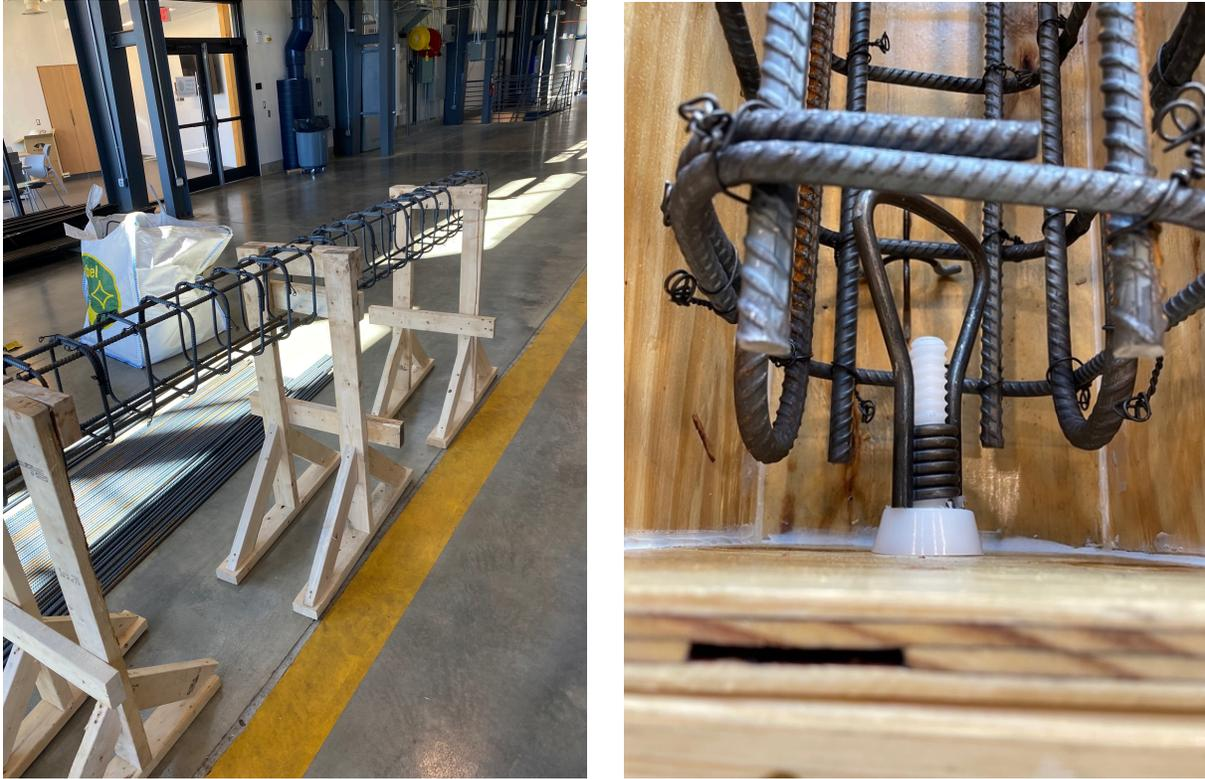
**Figure 5.6— Rebar Cage (left) and Lifting Hardware (Right)**
