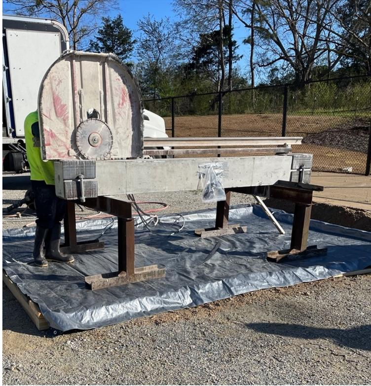
**Figure 7.7— Track Saw Mounted on Beam**
