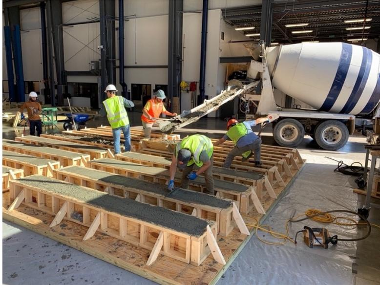
**Figure 5.9— Concrete Casting, Vibrating, and Finishing**
