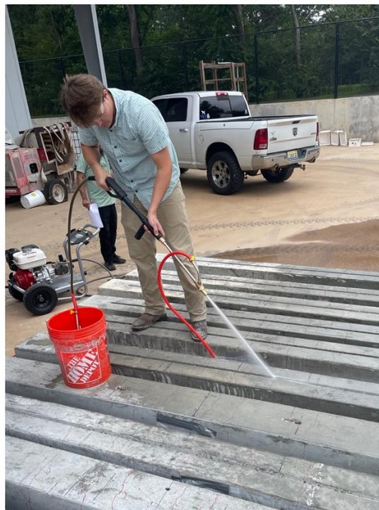
**Figure 7.10— Low-Pressure Water Blasting with Abrasives**
