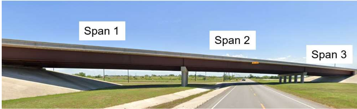
Figure 6-22. Chisholm Trail Bridge Spans
