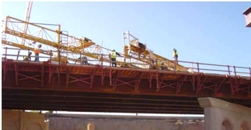
Figure 7-11. Lubbock Bridge During Deck Pour (Romage, 2008)
