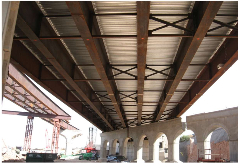
Figure 2-2. Lean-on Bracing in Lubbock, Texas Implementation Study (TxDOT Project 5-1772)
