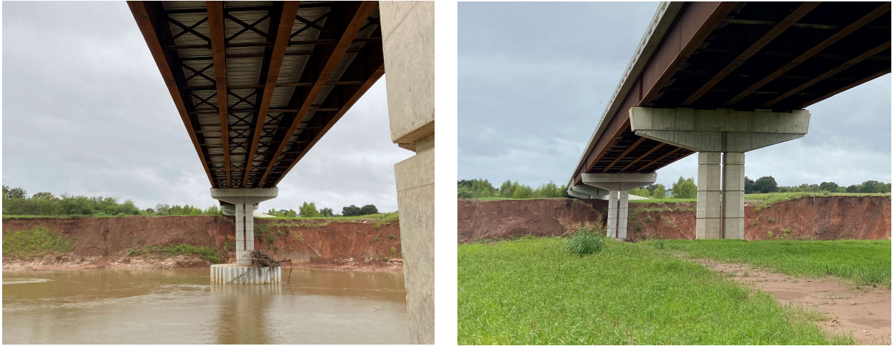
Figure 6-7. SH 105 Bridge Span 7-8
