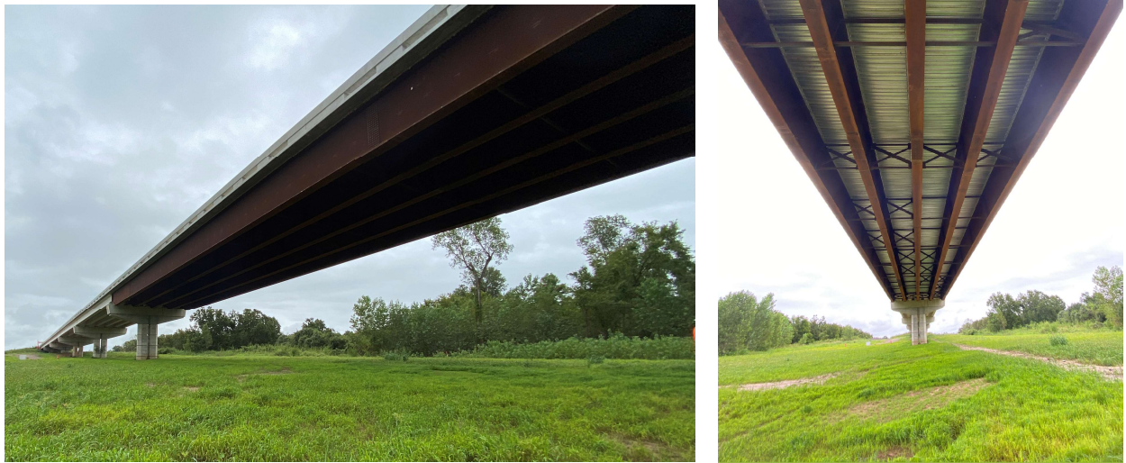
Figure 6-8. SH 105 Bridge Span 6
