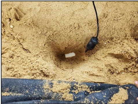
(a) Water content sensor installed in field sand
