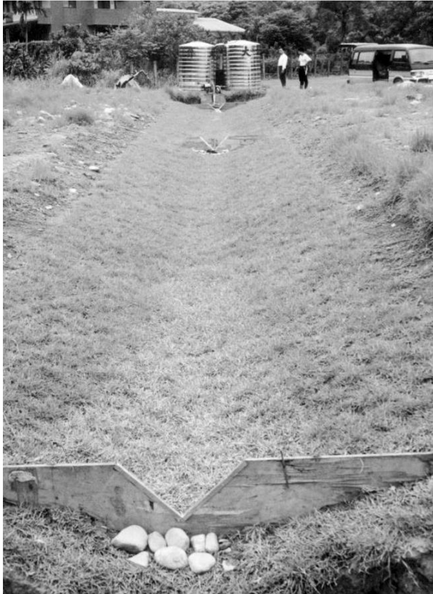
Figure 2-7. 32.8 yd (30 m) Swale with One Check Dam at Taiwan Test Farm (Yu et al. 2001).
