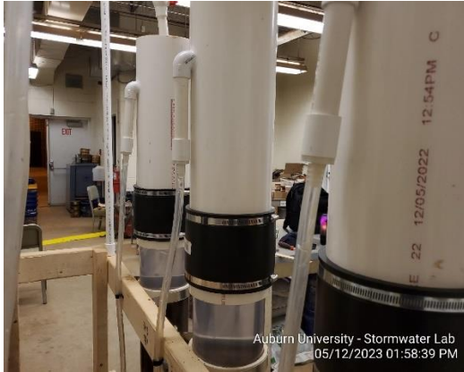
(a) Drainage system
