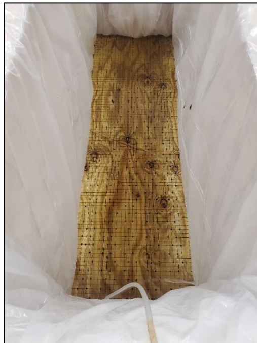
Figure 3-13. Plastic Sheetting and False Perforated Floor Installed.
